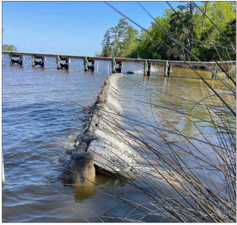
conditions and worked with Natrx on a digital design for custom ExoForm structures compatible with the permit requirements and that interlock with QuickReef™ units. Natrx helped advance the project from digital design, to physical production proof, to permit application and approval in less than one week. Natrx then produced 233 of the custom, naturalistic ExoForm structures to interlock with the Quick-Reef product, which Native Shorelines installed quickly and efficiently.
