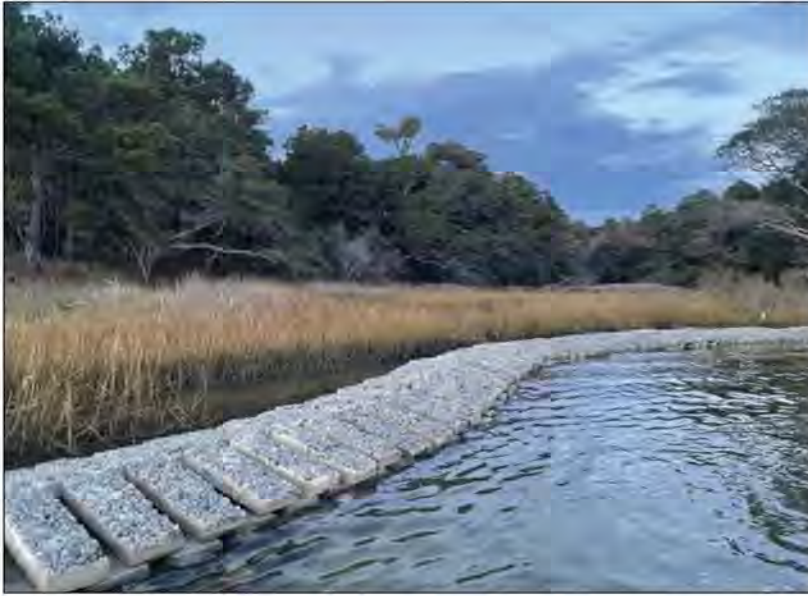
QuickReef is made from natural sources like limestone marl and oyster shells bound together with a small amount of cement.
