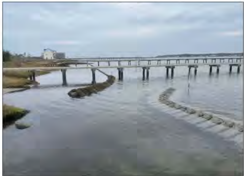
Living shorelines are arranged in shallow waters of the intertidal zone or can be designed as offshore sills.
