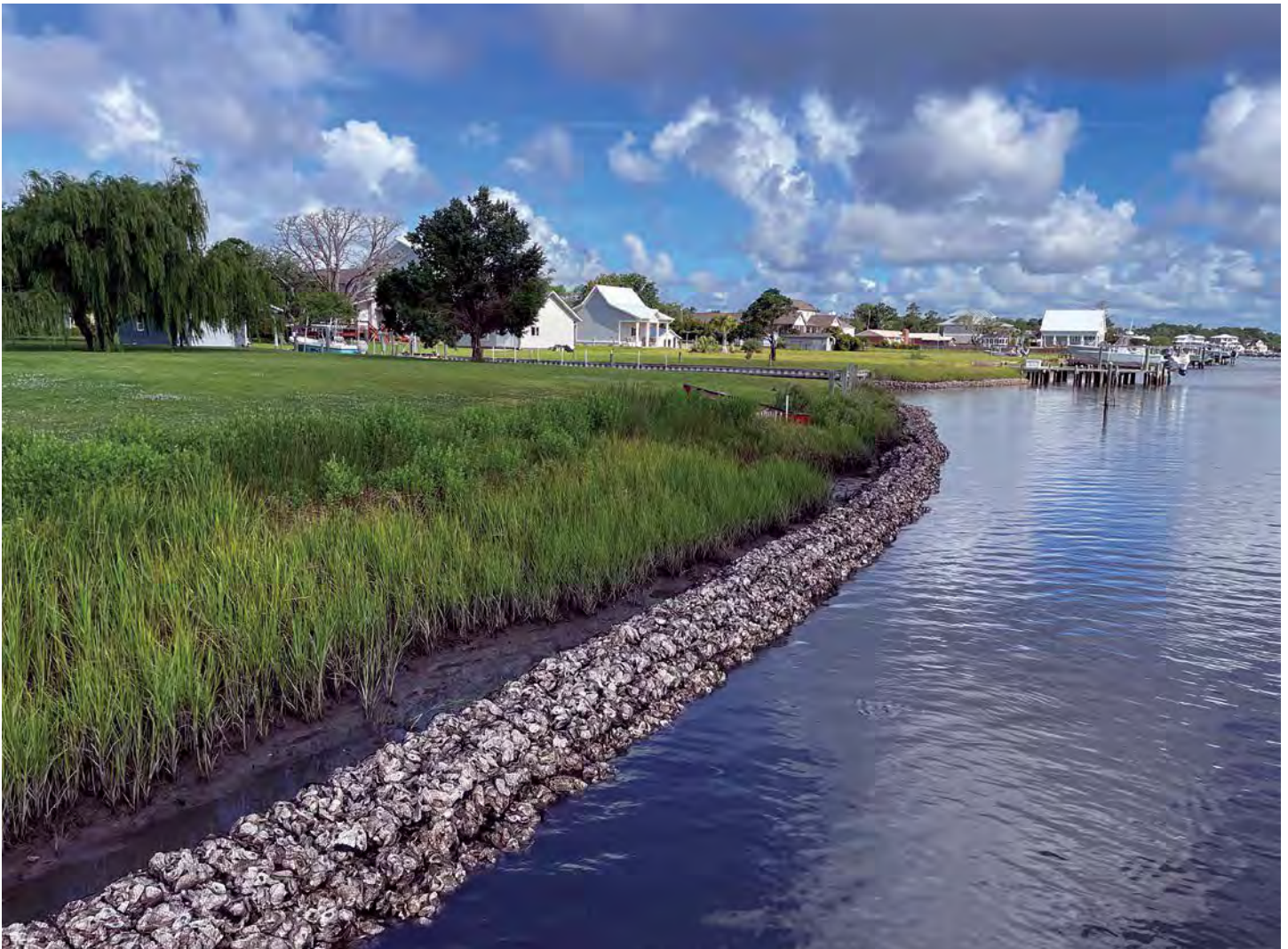
Oysters colonize quickly on QuickReef blocks, protecting the marsh behind them.
