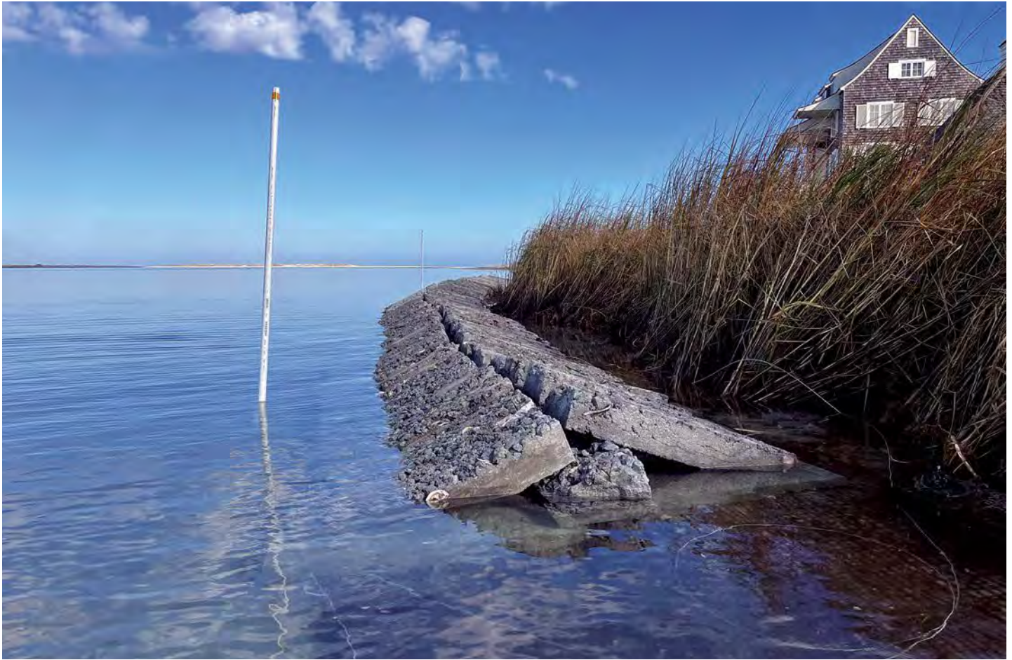
QuickReef blocks placed in the intertidal zone of a North Carolina bay.
